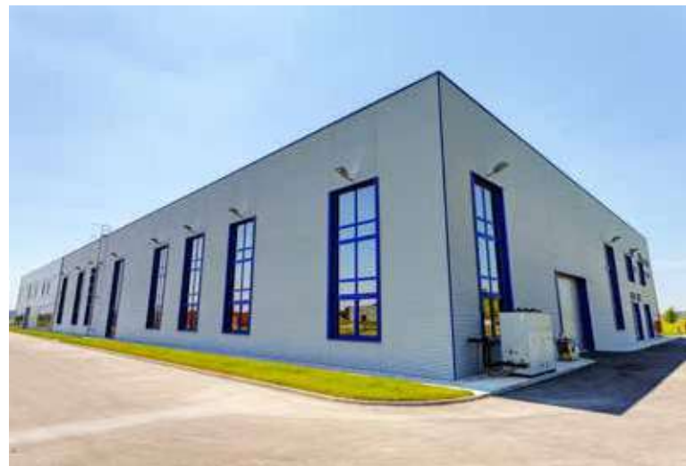
Air handling unit
