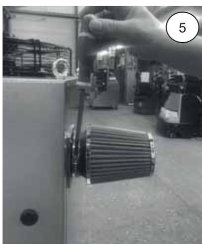
Tighten the air filter clamp with a screwdriver.
